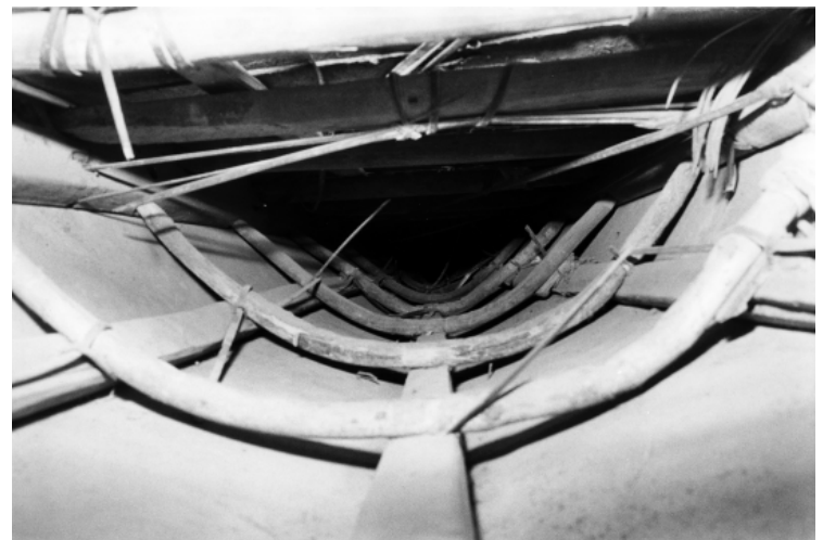
Figure 4.5 —Interior aft showing old deck beam lashing method.
